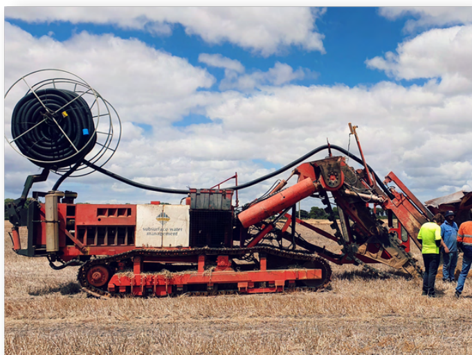
Subsurface drainage installation trial site. CREDIT: Ravensthorpe Agricultural Initiative Network.
