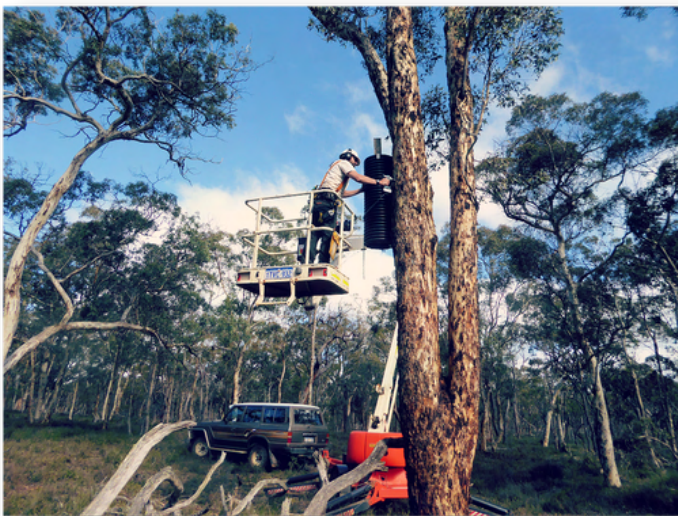
Installation of a Cockatube® at Balijup farm. CREDIT: Basil Schur, Greenskills.
