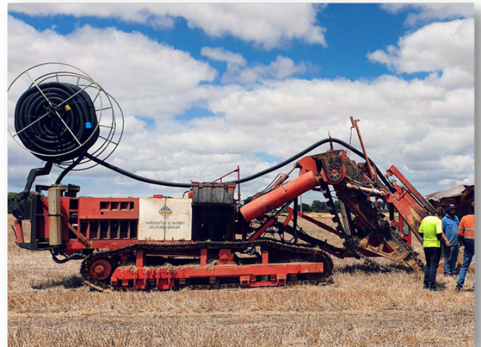
Subsurface drainage trial site. CREDIT: Ravensthorpe Agricultural Initiative Network.
